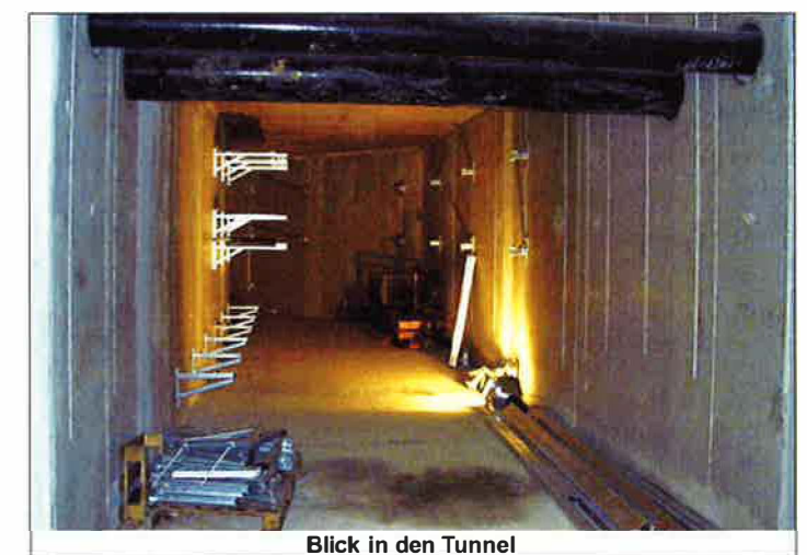
Blick in den Tunnel
